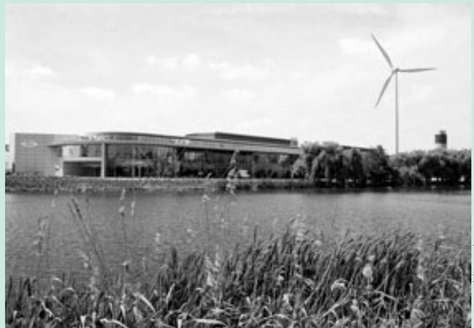
**One of the two 1.8 MW turbines powering Ford's new Dagenham Clean Engine facility. They generate over 6.7million kWh of electricity, which equates to supplying more than 2,000 homes.**
