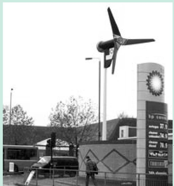
**A 6kW turbine providing power for a petrol station. The rotor diameter is 5.5 metres.**
