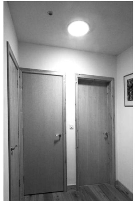
and two to bring more light into rooms. One is in a bedroom and can be darkened by bellows by means of a remote switch if you don't want to be woken too early.
