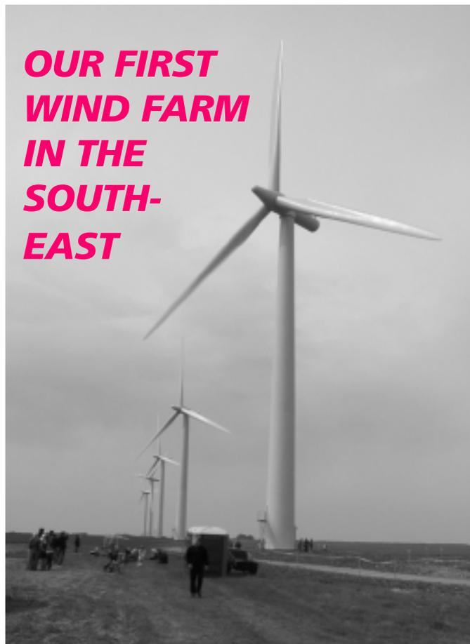
arrived on site at 0830 and the turbine was fully erected the same day at 1830. The 49m towers come in two sections each weighing about 25 tonnes, the nacelles each weigh 50 tonnes and the rotors 30 tonnes.
